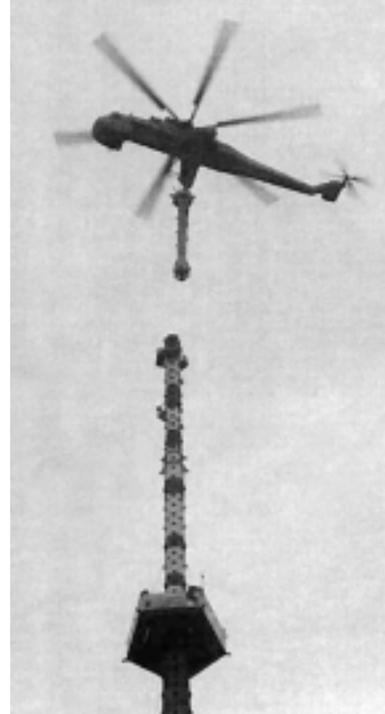
commissioned to assemble the Tower's antenna, the slim, stacked broadcasting receptor rising 350 feet from the shaft. Before it could start lifting pieces of the antenna into the sky, the helicopter dismantled the crane in eight sections. After that, Olga lifted the 36 pieces of the antenna into place with remarkable precision. As the helicopter raised each piece of the antenna, fearless workers helped manoeuvre and bolt the new piece into place in gusting winds and
