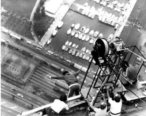
24 hours a day, five days a week, concrete was poured into a massive mold or "slipform". As the concrete hardened, the slipform, supported by a ring of climbing jacks powered by hydraulic pressure, moved upwards, gradually decreasing in size to produce the Tower's gracefully tapered contour.
