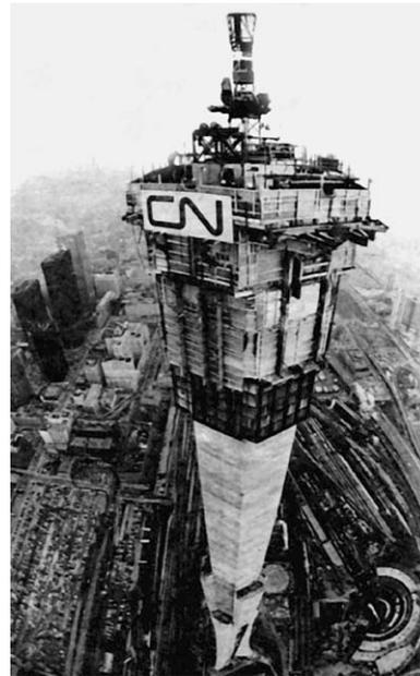
The radome (the donut-shaped collar at the base of SkyPod), protects the Tower's sensitive microwave equipment and is essential to its intrinsic purpose as
