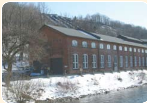
Decew Falls original building. IEEE Hamilton Section
