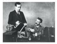
At Signal Hill on December 12, 1901, Guglielmo Marconi and his assistant, George Kemp, confirmed the reception of the first transatlantic radio signals. With a telephone receiver and a wire antenna kept aloft by a kite, they heard Morse code for the letter "S" transmitted from Poldhu, Cornwall. Their experiments
