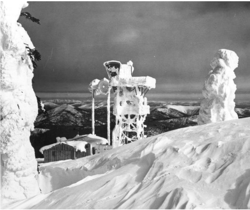
A Trans-Canada microwave relay station on a mountaintop near Creston, B.C., 1959
